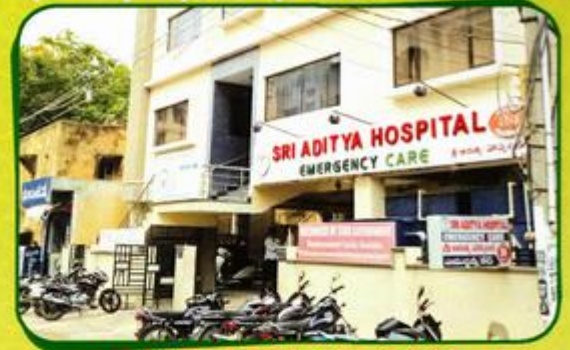
SRI ADITYA HOSPITAL RAJAHMUNDRY
